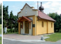
the Chapel in Kornicy
